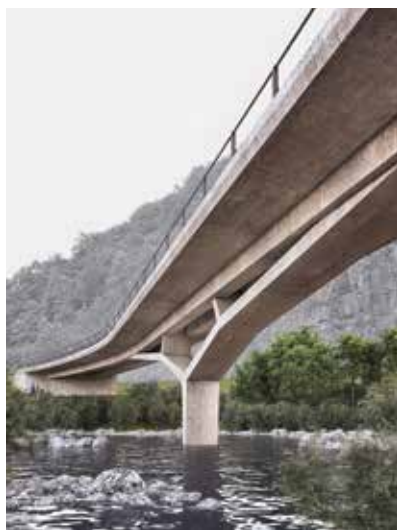
Ponte Sassello, Roveredo
